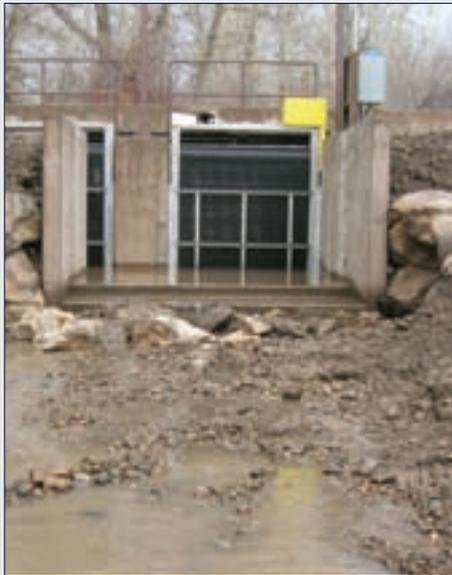
The Hydrolox screen now prevents fish from entering the irrigation canal.
